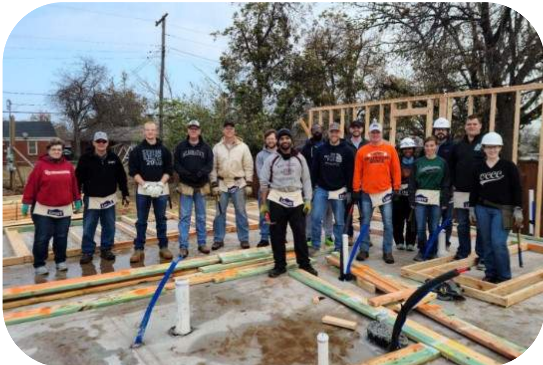
Habitat for Humanity House Framing Work Day
