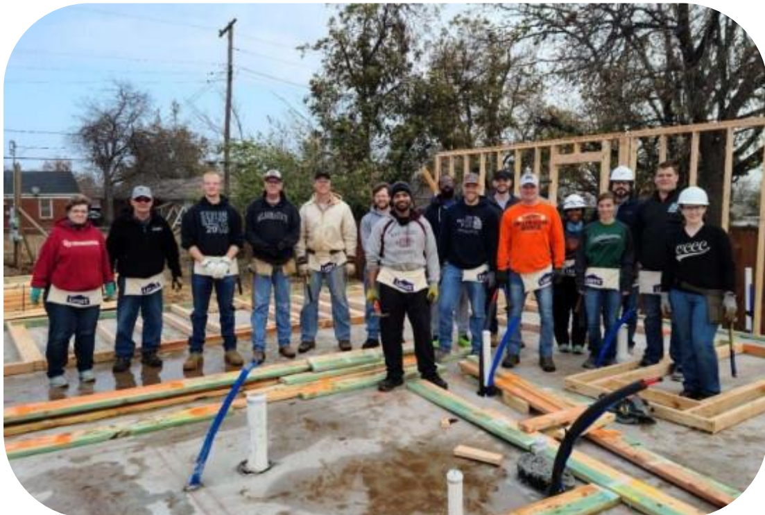
Habitat for Humanity House Framing Work Day
